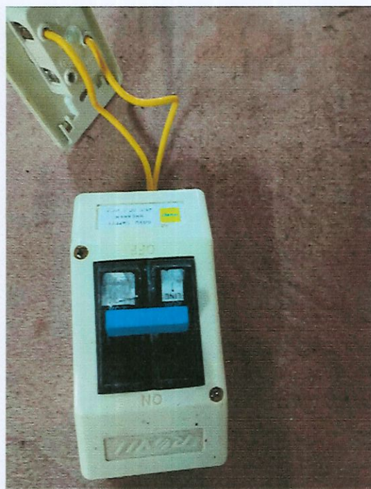
Circuit Breaker Switch 30 ampere with Housing
