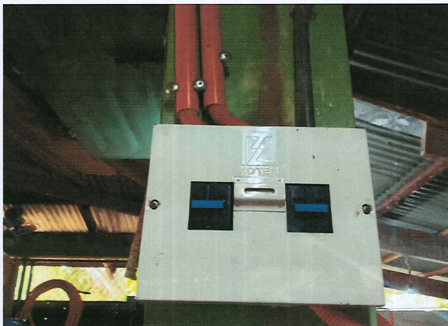
Double Throw Switch Breaker Type 100 Ampere
